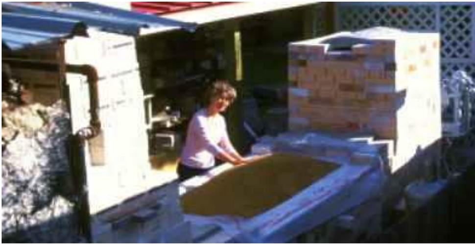
Carol putting finishing touches on sand mould for inside contour of castable firebrick lid. Note firebox height and the underside of the castable arch which tops the firebox.
