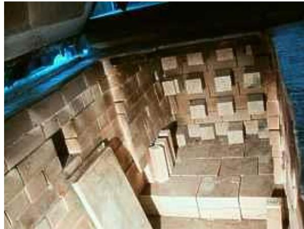
Checked exit flue with "damper" plugs for firing old kiln. Note step up of floor and narrowing of the tail to 27 inches. Also note backstoking hole on left.
