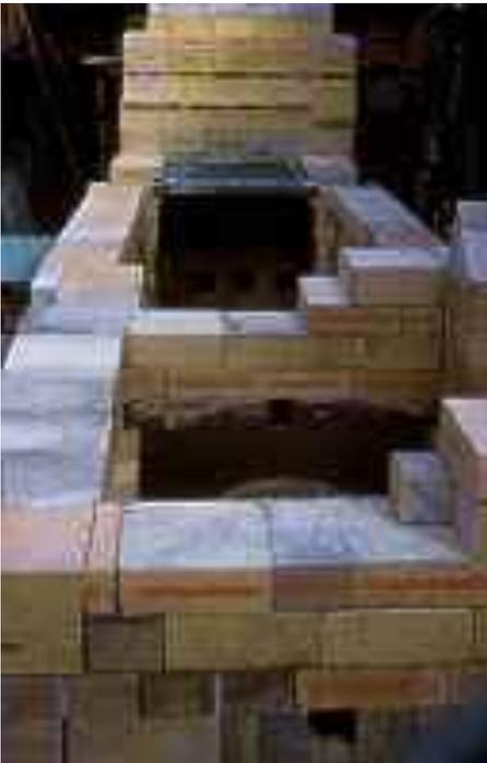
View from firebox through the throat arch and main chamber and chimney.
