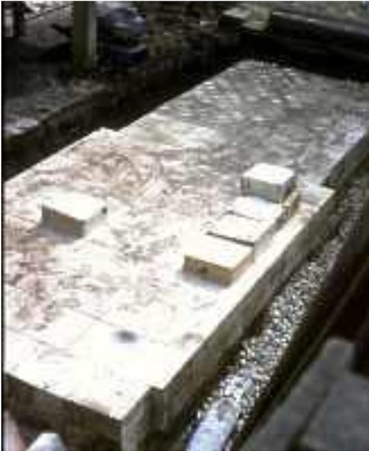
8 inch firebrick floor on top of 5 ½ inch cast able on top of 5 1/2 inch concrete foundation. Note the weeping tile and gravel around the foundation. The floor is at ground level with the first 2 feet of the kiln in the ground
