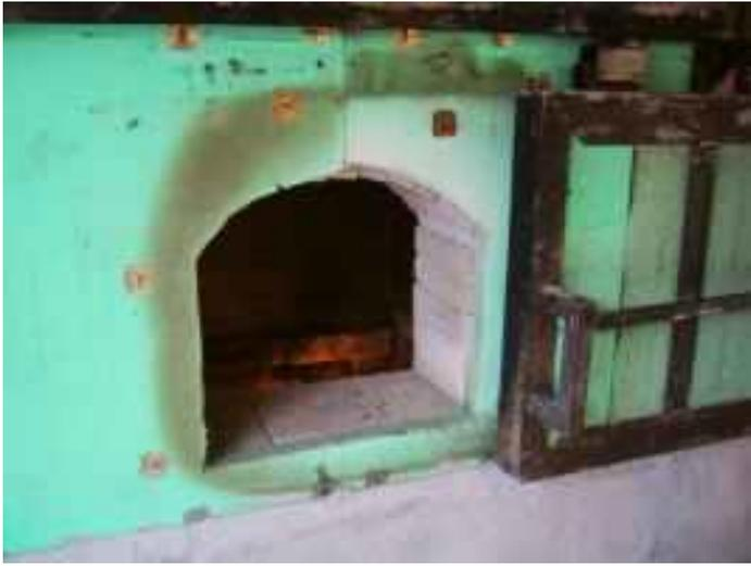
Block insulation on metal pins with open door.
