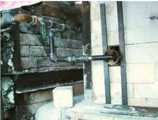
Gas after-burner in chimney above damper. This may require a small blower to provide more oxygen. Pipe union allows for removal of burner.
