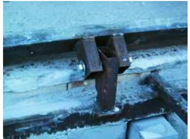
Detail of hinge mechanism welded to lid and frame.
