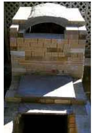
Shelf top and insulator bricks with castable over tumble stack area
