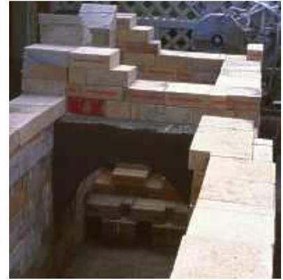
Cast throat arch and step grate in firebox. Note width of kiln increases to 31 1/2 inches after 27 inch firebox and first throat arch tumble stack firing area
