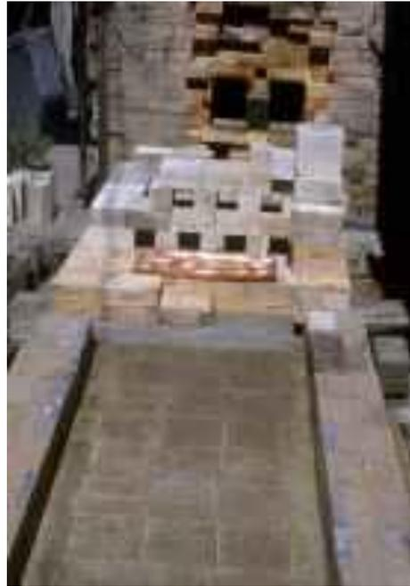
Start of checkered exit flue at the base of the new chimney, which serves both kilns Note the exit flue from the old gas and woodfired two chamber kiln.
