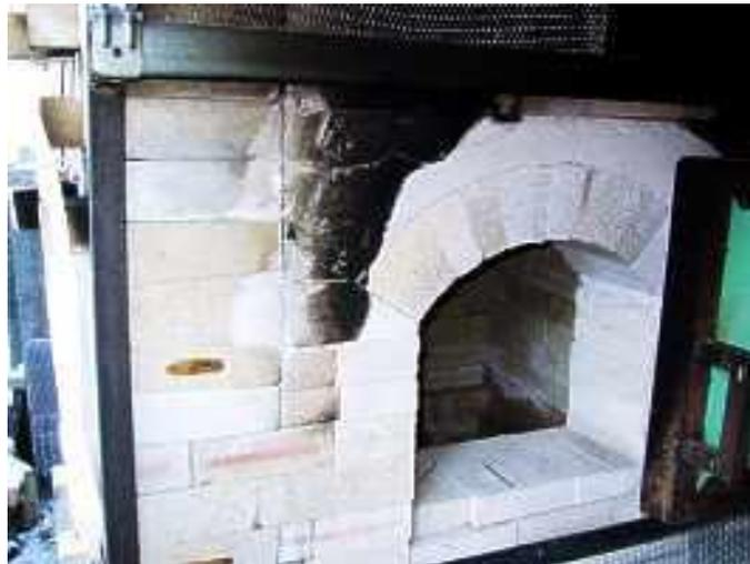
Hansel and Gretel firebox stoking door before the addition of block insulation . Note barn door hardware for sliding door.
