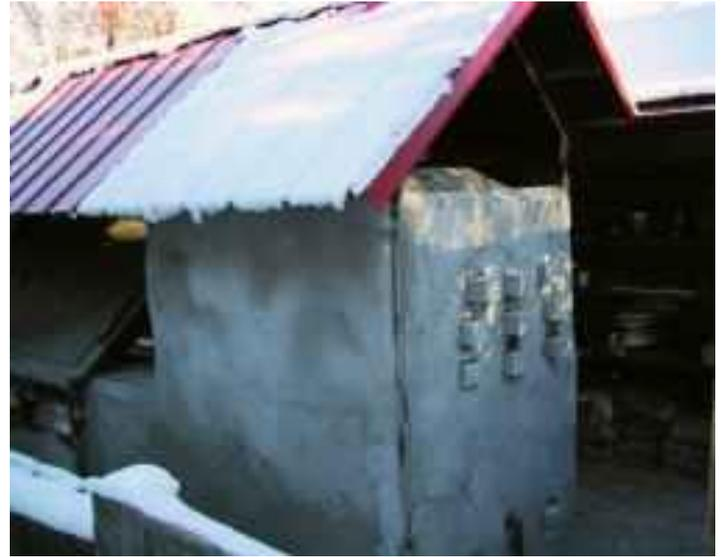
Elevated firebox with intake air holes plugged.
