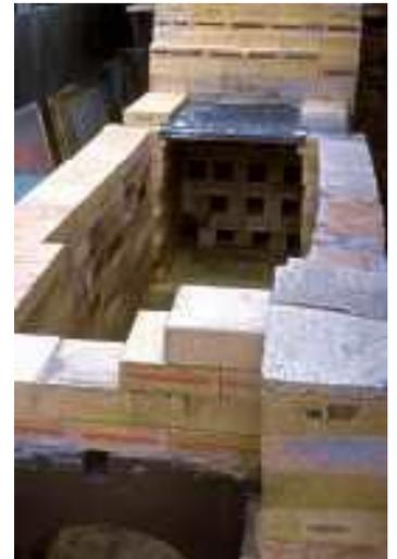
Checked exit flue with plugs removed Note 28 inch silicon carbide kiln shelf that acts as top for tail section.
